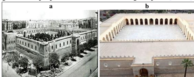
Figure (1) general view of the Al-Zahir Baybars Al-Bandaqdari mosque in Cairo; a. before restoration, b. after conservation processes
