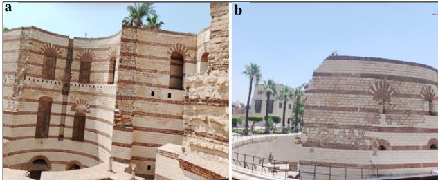
Figure (2) a. remains of the Roman tower guarding the Roman canal, b. exterior of the Roman tower that flanked the entrance to Trajan's canal.
