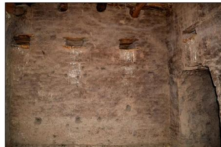
Plate (12) tabia S. wall of ground floor
