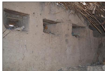
Plate (35) tabia W. wall of the ground floor
