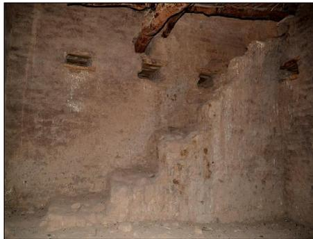
Plate (13) tabia eastern wall of ground floor
