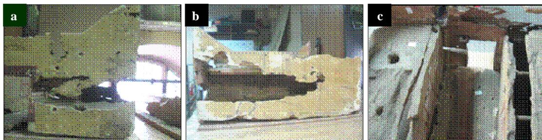
Figure (10- a, b, c) deterioration of wood (weakness in the bonding forces between fibers), and fungi infection.
