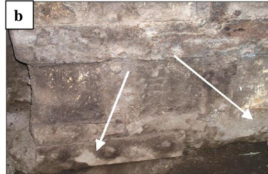
Figure 11 (a, b) deterioration phenomena on Overlaid wooden door of Ibrahim Sarhan caravansary
