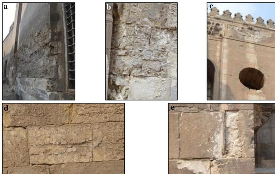
Figure (3) Shows weathering phenomena of the limestone used in Qaytbay mosque **a.** **b.** lower parts, **c.** upper parts, **d.** and **e.** middle parts of the mosque walls
