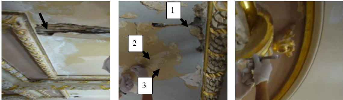
Figure (1) Show a Separation of all layers from the wooden support in the ceiling of Abdeen Palace, b samples from the paint layer Of Abdeen Palace:1= green colour,2= creamy yellow colour, 3= brown colour, c the gilded parts Of the ceiling Of Abdeen Palace.
