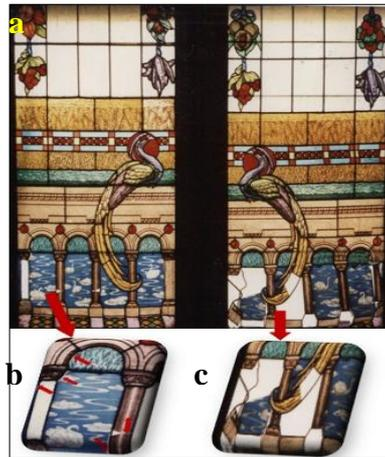
Figure (3) Shows **a**. lead net is weak as it is greatly unable to keep the panel in the up-right position, **b**. cracks and illumination of the glass, **c**. breaking the welding and losing of glass pieces as a result of the weakness of the lead net.
