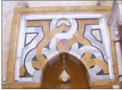
Plate (6-f) Shows the upper part of the mihrab, overlapping circles formed the voussoirs of the pointed arch.
