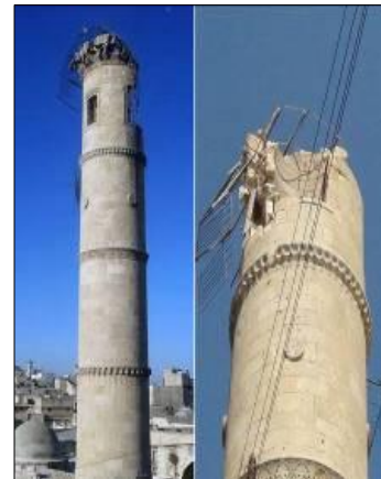
Plate (4-d) Shows the destroyed part at the top of the minaret during the current events in Syria
