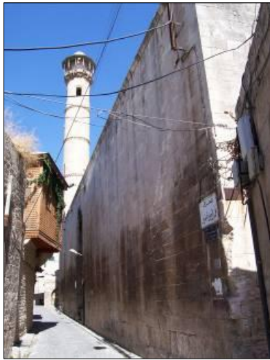
Plate (2) Shows the northern façade of the mosque, the main façade.
