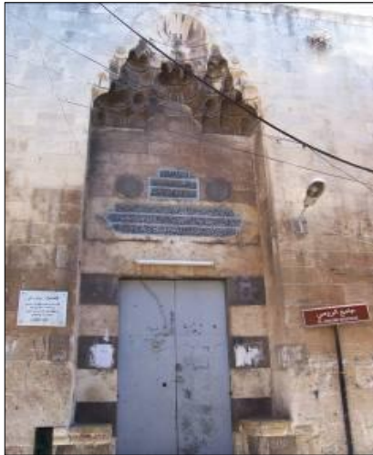
Plate (3-a) Shows the main entrance of the mosque
