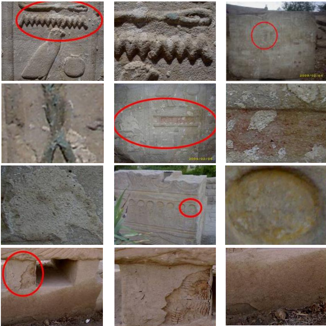
Fig.9 (a-l) Show the same colored relief sandstone Stella "the case study " suffering from different aspects of deterioration in details" notice the deteriorated wooden beams".
