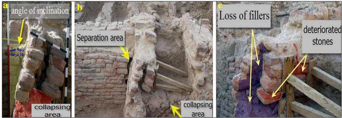
Figure (4) Shows **a.** inclination angle of the wall, **b.** separation and collapsing areas, **c.** loss of internal fillers and stone deterioration
