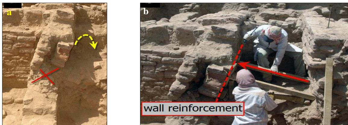
Figure (3) Shows **a**, tending wall after discovering, **b**, diagonal and horizontal reinforcement
