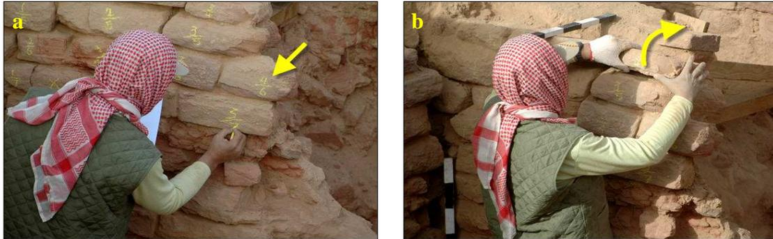
Figure (10) Shows **a.** stones numbering, **b.** beginning of the manual loosening processes
