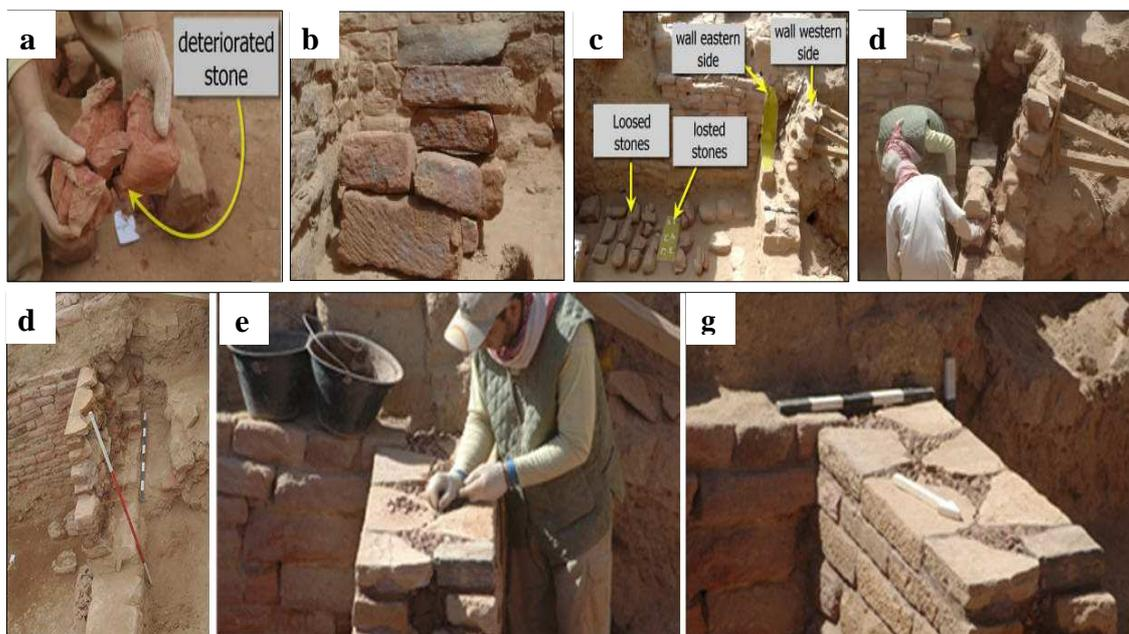
Figure (12) Shows **a.** sample of deteriorated stones after loosening, **b.** examples of alternative stones, **c.** removing the tending part of the western side, **d.** the beginning of rebuild, **e.** removing the tending part of the western side, **f.** small gravels were fixed on the filling layer surface to distinguish restored part, **g.** Dedan wall after conservation
