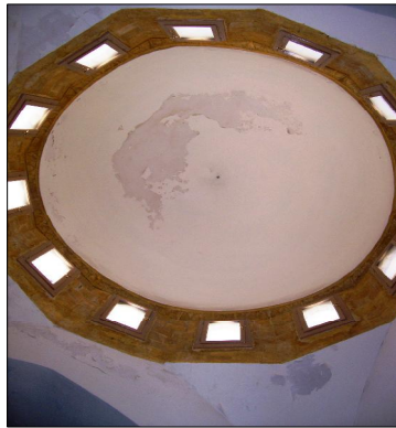
Plate (9) The dome in front of the Mihrab from inside
