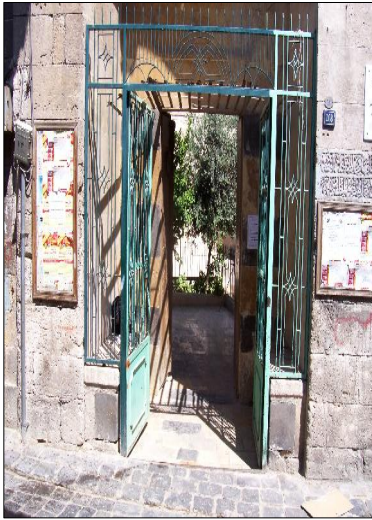
Plate (2) Lower part of the main entrance
