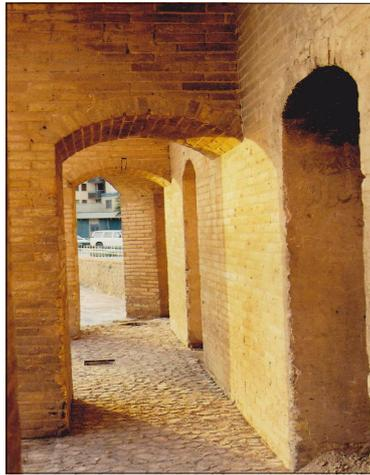
Figure (8) the segmental and half arches used in bridges' corridor
