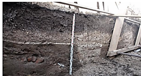
Figure (7) Shows section of the foundations and the lime floor (After: Hawass Archive, 2010).
