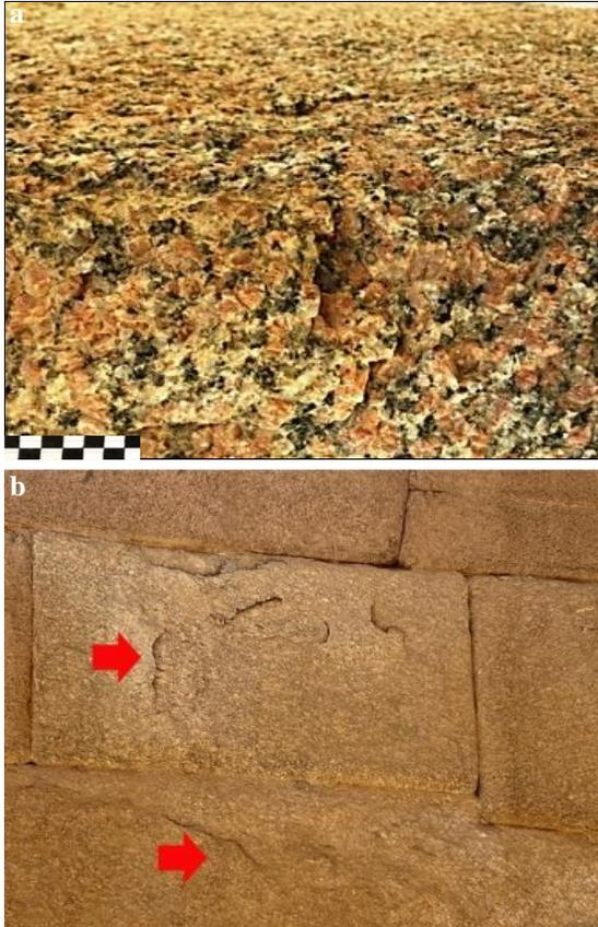
Figure (5) Shows **a.** the different minerals that make up granite **b.** separation in layers due to the variation in the physicochemical composition of the granite minerals
