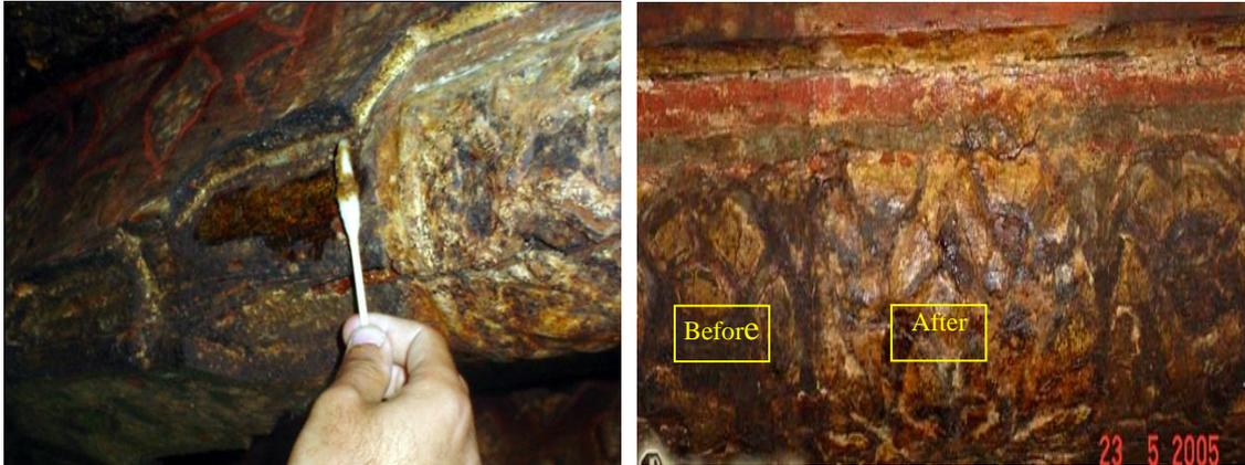
Figure (18) the chemical cleaning of the painted ceiling.
