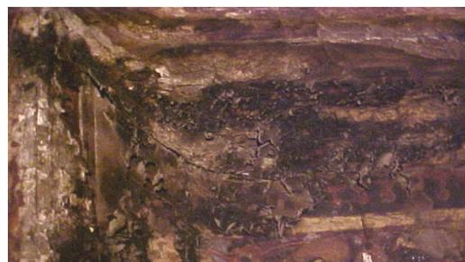
Figure (10) microbiological infestation causing discoloration often associated with detachment of the paint layer.
