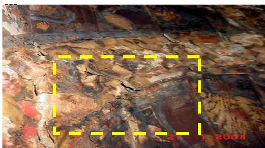
Figure (9) crumbling in some parts of plaster.
