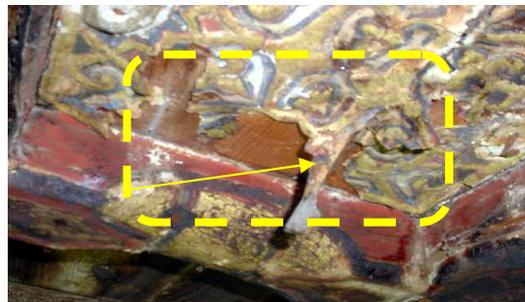
Figure (4) separation of painting layer of the ceiling.
