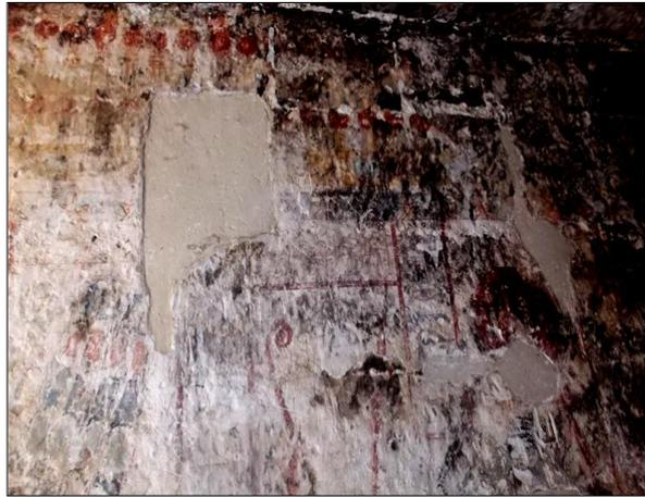
Figure (6) Shows the humidity impacts on the walls of archeological sites under investigation
