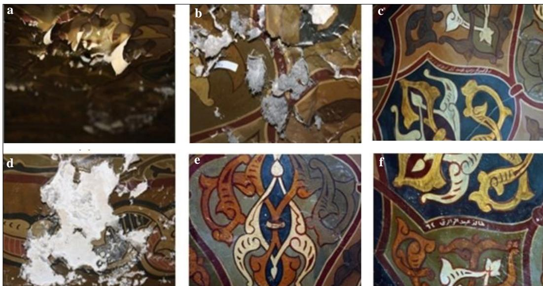
Figure (2) Shows examples of deterioration phenomena of the painted dome **a.** flaking, detachments, **b.** salt weathering, **c.** Conservator's signature, **d.** missing areas, **e.** & **f.** darkening and over-painting
