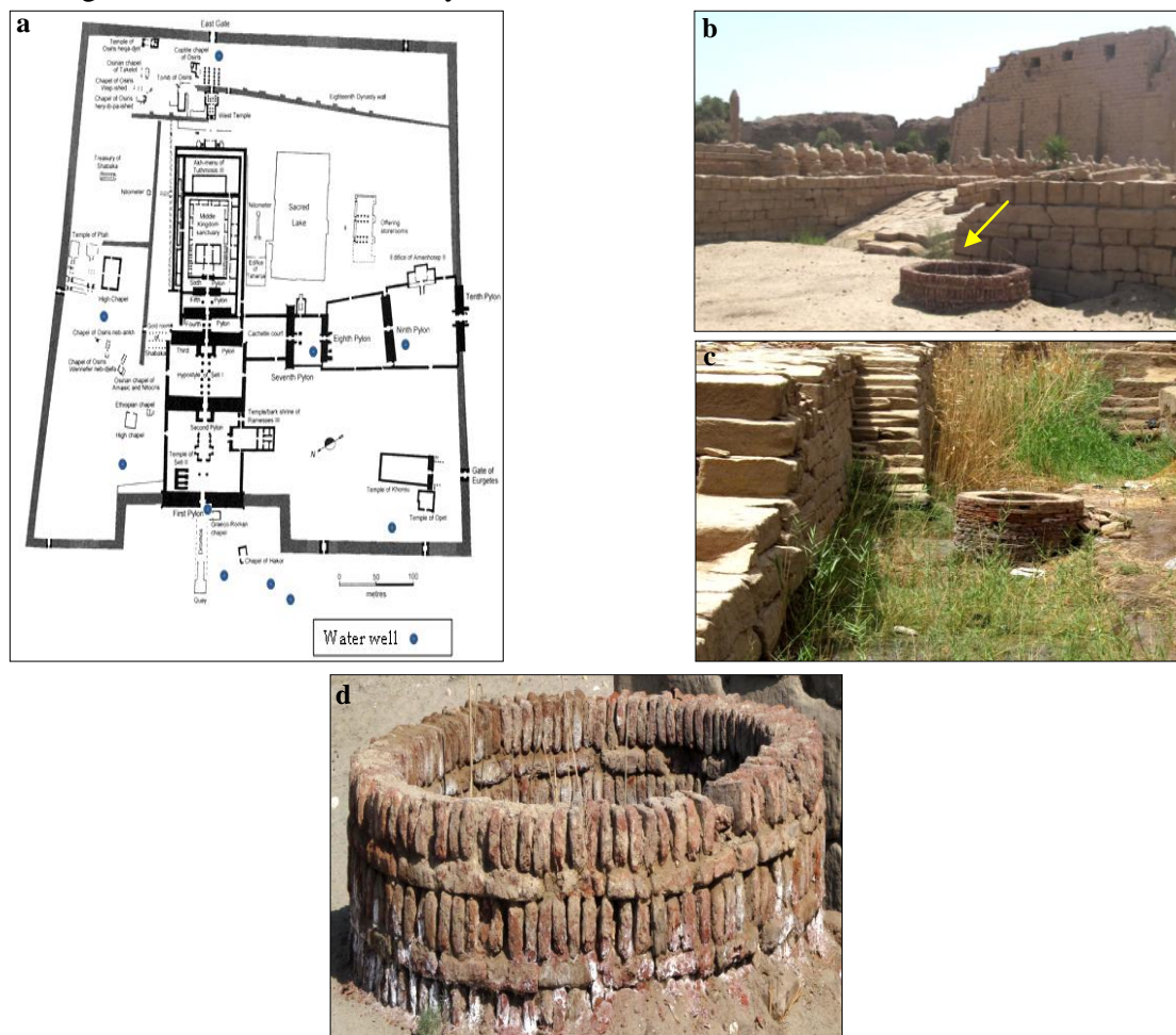
Figure (1) Shows a. location of water wells inside Karnak temples complex (after Blyth, 2006 & CNRS 2019), b. well in the front of the first pylon of Karnak, c. well close to embankment at El-madrassa site, d. building methods of water wells at Karnak temples
