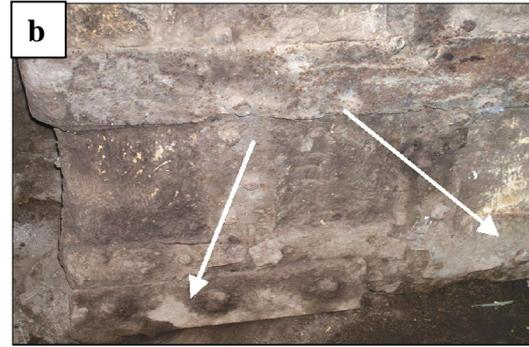
Figure 11 (a, b) deterioration phenomena on Overlaid wooden door of Ibrahim Sarhan caravansary
