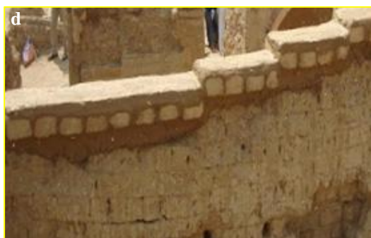
Figure. (11) Shows a , applicable technique for prop up the cracked/damaged shrines, b , a model for covering by shelters and capping method carried out by the researcher in a similar adobe building c , application of plastic sheets, d , protective courses.
