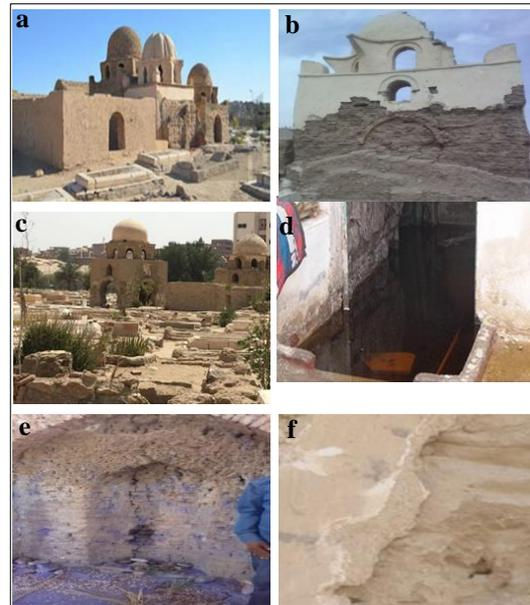
Figure (2) Shows **a**, some different forms of domes in the Fatimid cemetery in Aswan, **b**, fall off of small and large pieces of plaster, **c**, fall of the plaster layers, as well as the trees and plants **d**, accumulation of saline groundwater in the tomb of Sidi Abdel Aal, **e**, blue pigment that distorts the walls and covers the floor of the Sharia judge's cemetery, **f**, fall of the plaster layers with the pigments above from the tomb of the Sharia judge.
