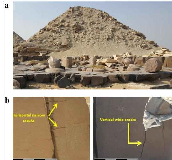
Figure (1) Shows **a.** remains of basaltic walls and pavements in the temple of Niuserre at Abu Sir, **b.** horizontal and vertical cracks affected the basaltic walls
