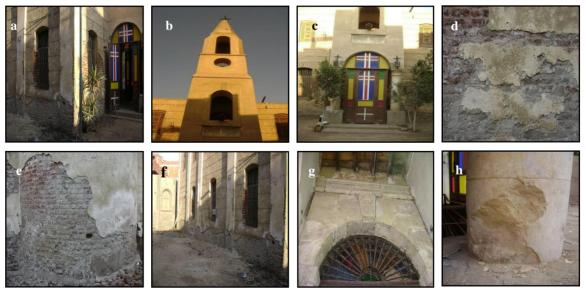
Figure.(2) <u>a</u> deterioration of walls, <u>b</u> the tower, <u>c</u> the church entrance, <u>d</u> damage of brick units, <u>e</u> decay of plaster layers, <u>f</u> rising damp in the walls, <u>g</u> crystallization of salts on stone surfaces, <u>h</u> missing parts from one of stone column.
